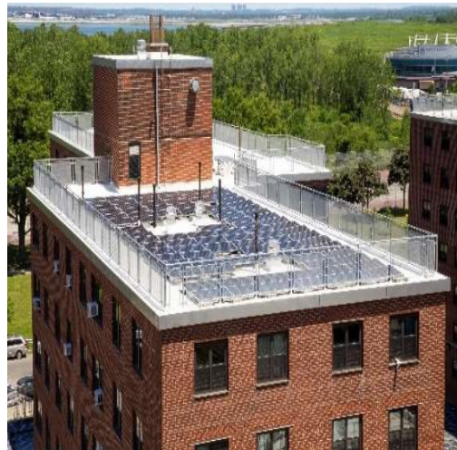
Repaired roof and solar panel system at Ocean Bay (Bayside)
